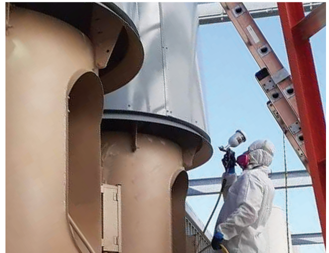
HVAC NEW LIFE PROCESS
