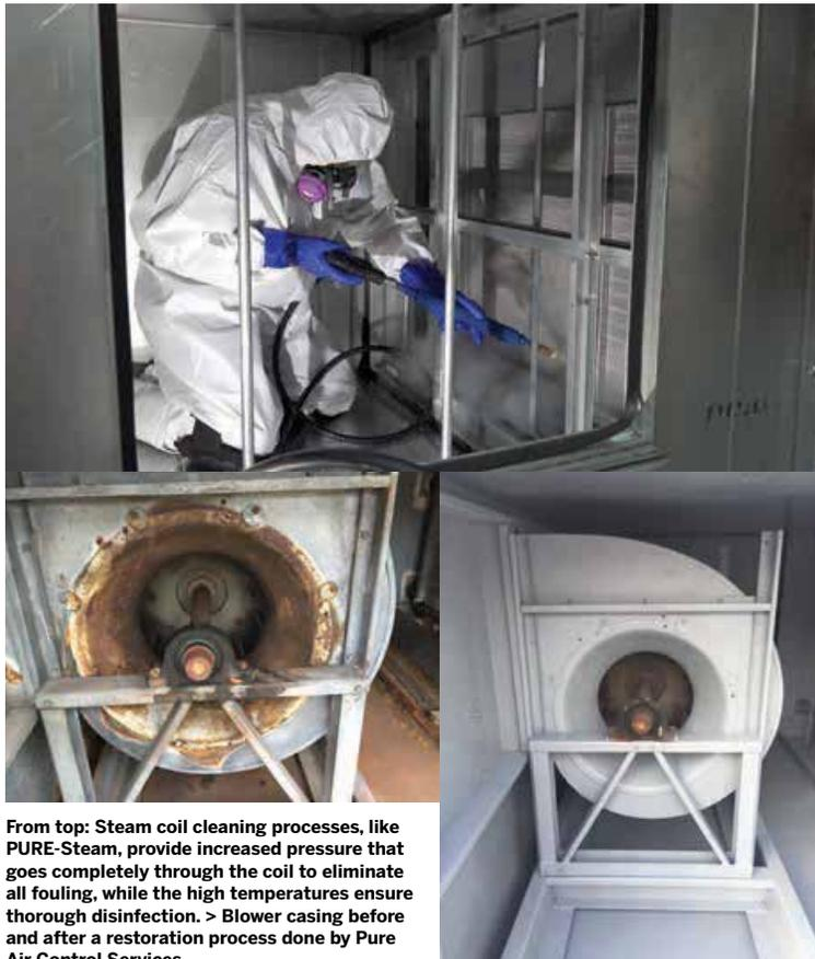
From top: Steam coil cleaning processes, like PURE-Steam, provide increased pressure that goes completely through the coil to eliminate all fouling, while the high temperatures ensure thorough disinfection. > Blower casing before and after a restoration process done by Pure Air Control Services.
