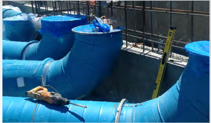
DUCT Work Underground - PURE-Liner Blue
